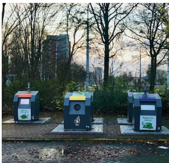
Picture 29: Streetside residue bins in Amsterdam, classified by color for each material. The large bins are situated underground. December 11, 2021. Photography by Carmen Rial.
