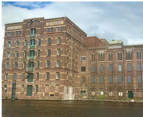
Picture 4: Old factory on the banks of the Zaan River. September 2019. Photo by Cornelia Eckert.
